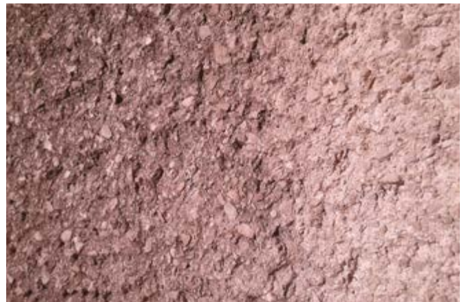
Friable and worn out surface
