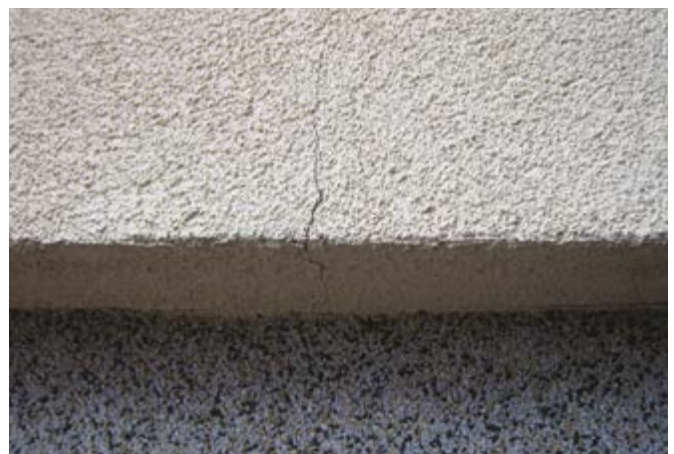
Static damage
